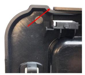
3. Remove 0.7 mm from the upper tab (arrow) using a file. A feeler gauge can be used (shown lying flat along top edge) to assist with measuring.
