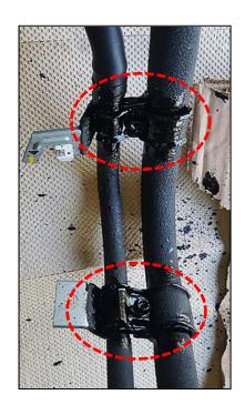
15. After spaying, tie the CCV wiring and vent pipe using band strap (O).
