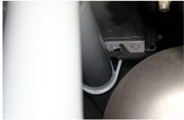
FIGURE 99: ENGINE INTAKE PIPE SUPPORT
