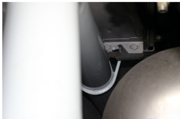
FIGURE 96: ENGINE INTAKE PIPE SUPPORT
