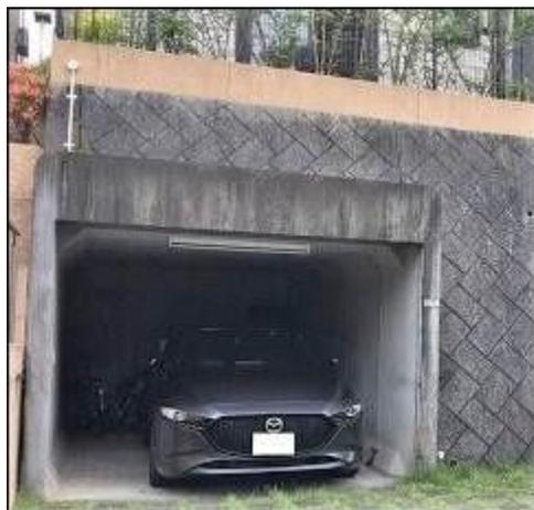
This concern may be caused by refraction and/or diffraction of the signal used for the advanced keyless entry system by the steel reinforcement bars in the concrete walls. As a result, the signal will resemble a theft attempt (known as a Relay Attack) and the anti-theft function of the advanced keyless entry system will prohibit door lock operation. To eliminate this concern, the LF control unit software has been modified to reduce the improper detection of the theft attempt.
