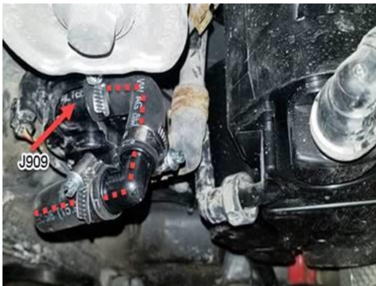
Figure 9. Closer look at the connections.
