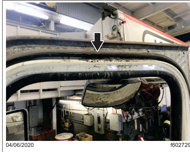
Fig. 2, Road Grime on Door Seals
