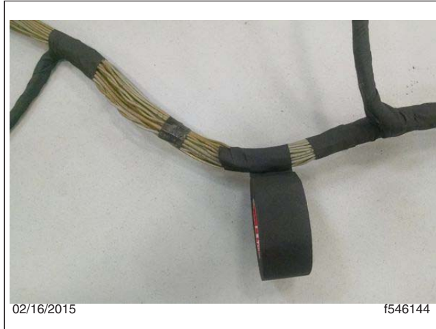
Fig. 14, Wrapping the Harness with Fiber Tape
