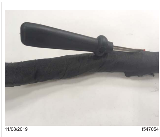
Fig. 9, Cutting an Opening into the Fiber Wrap
