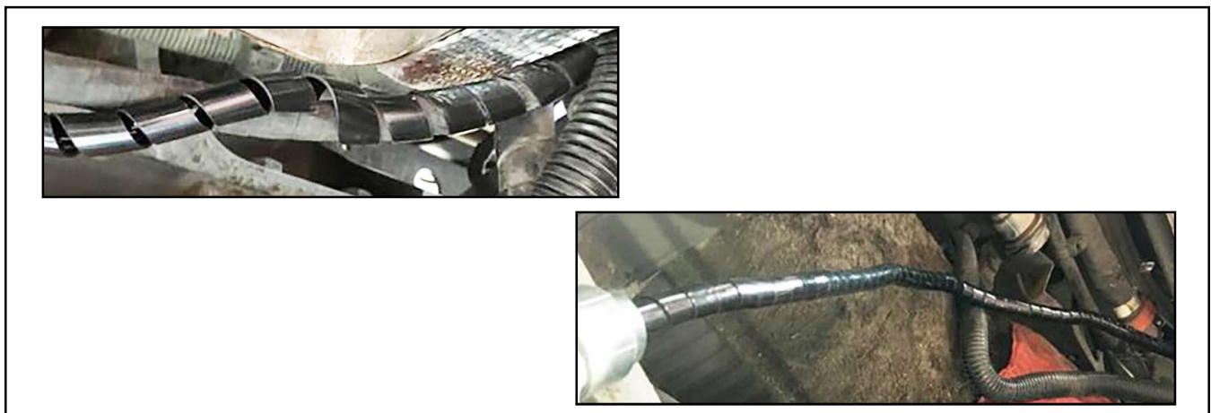
Figure 6 - Spiral Sleeving Installation
