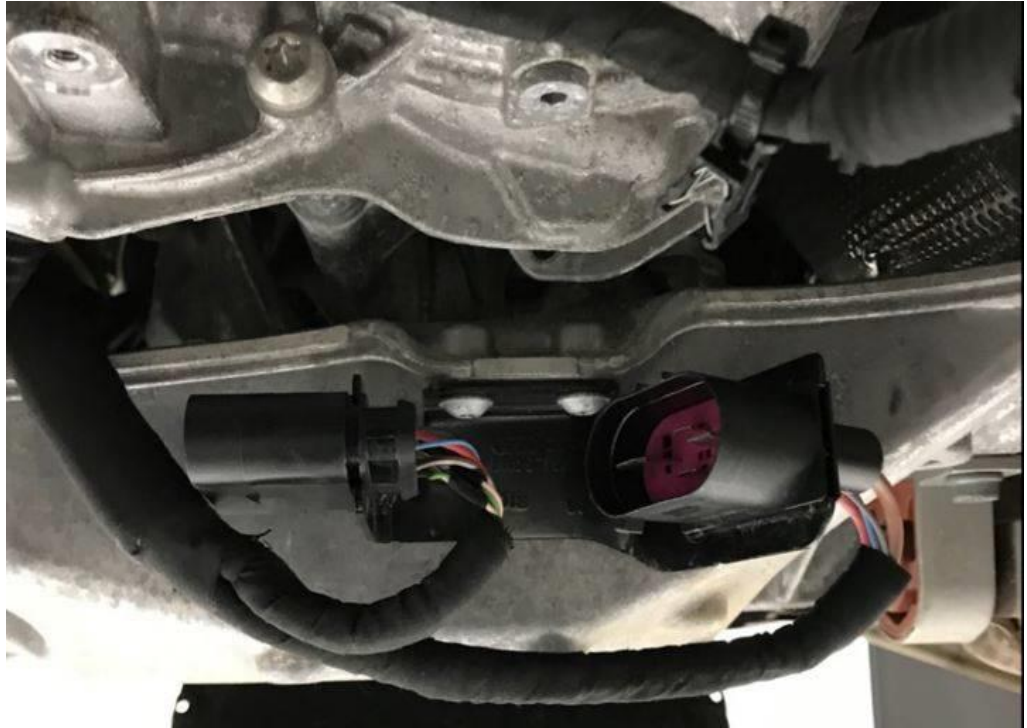
Figure 14. New transmission harness routing.
