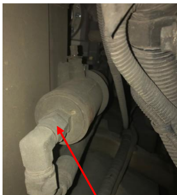
Power steering pump supply line
