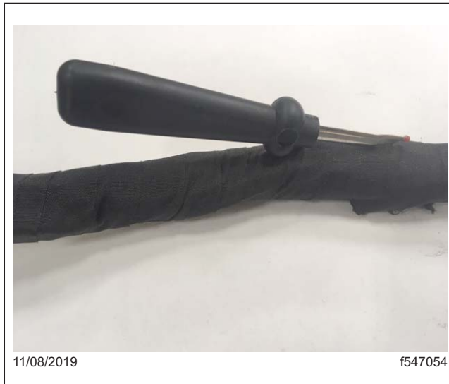
Fig. 9, Cutting an Opening into the Fiber Wrap
