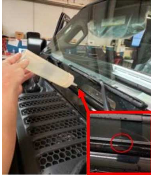
Fig. 1 Inspect for Leaks
