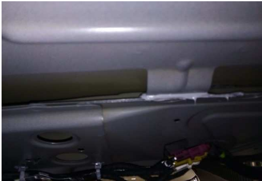
Fig. 3 Sealant Applied To Repair Area
