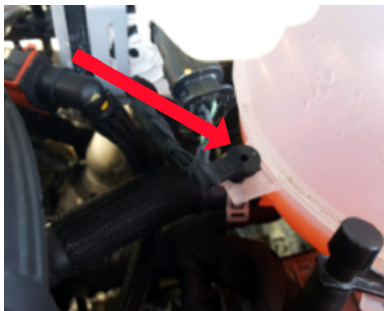
Above shows the brake fluid level sensor correctly connected.
