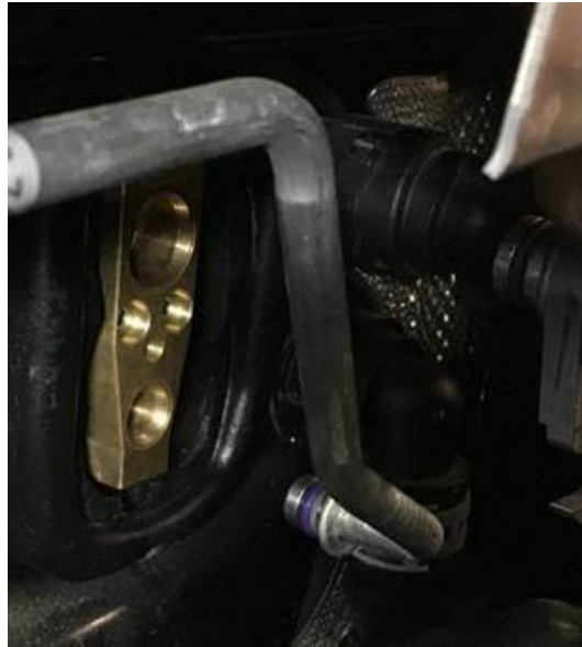
Figure 3. Installation of front expansion valve bypass adaptor VAS 6338/38.
