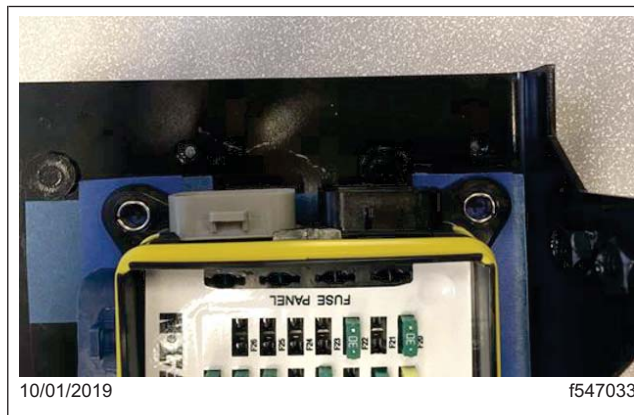
Fig. 3, Using the new PDM to Mark Drill Holes
