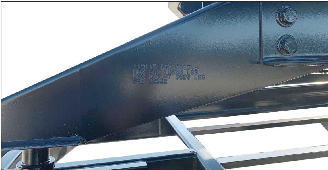
Fig.3 Dot Peen After Powder Coating
