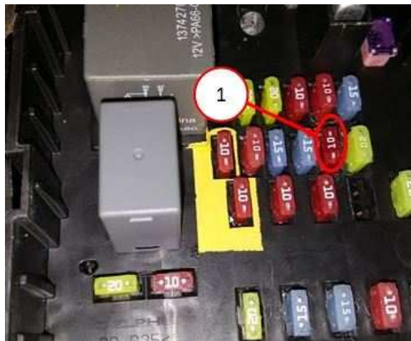
Fig. 10 JC Fuse Panel
