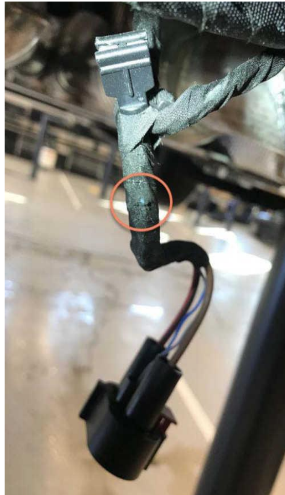
Figure 3. The damage on the harness might be difficult to spot.
