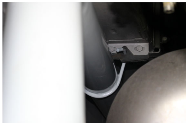
FIGURE 99: ENGINE INTAKE PIPE SUPPORT
