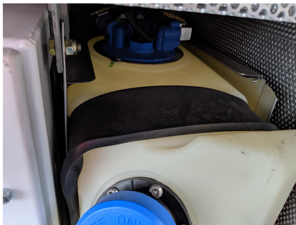
Incorrect Strap Orientation
