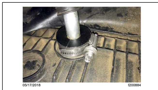
Fig. 7, Collar and Clamp Installed
