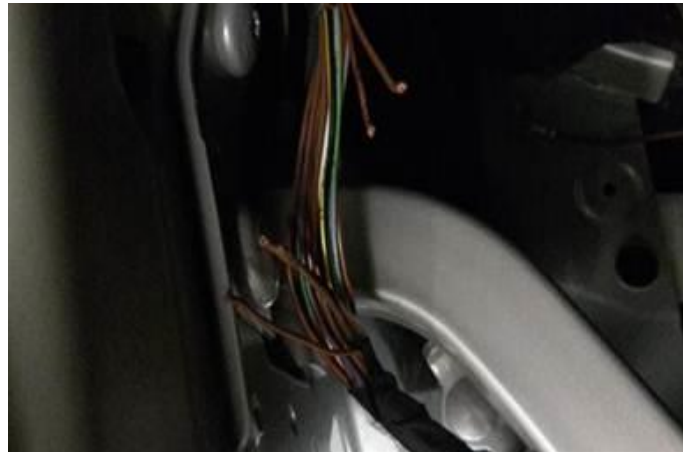
Figure 1. Wire damage at the trunk hinge.
