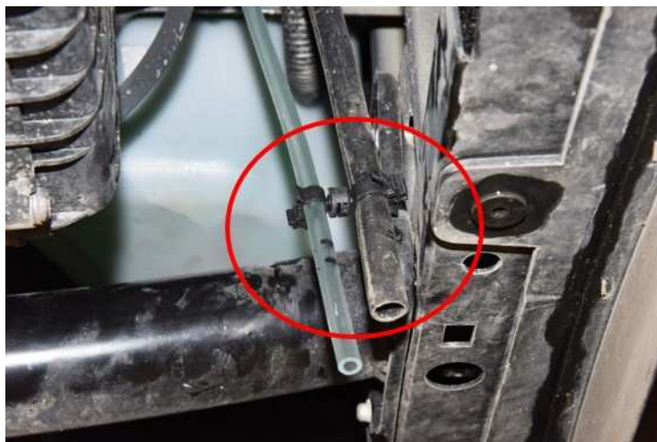
Fig. 18 Clamp Installed On Hoses
