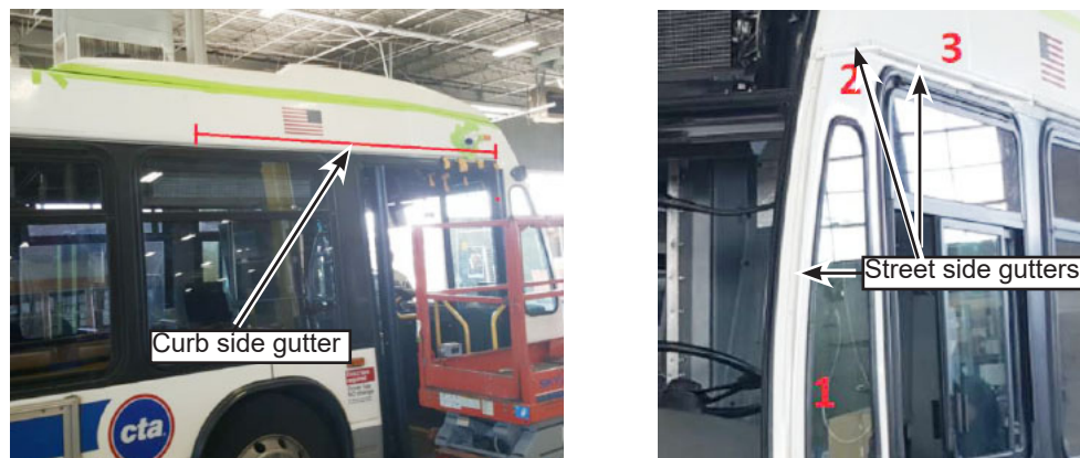
Figure 43 - Install the Gutters
