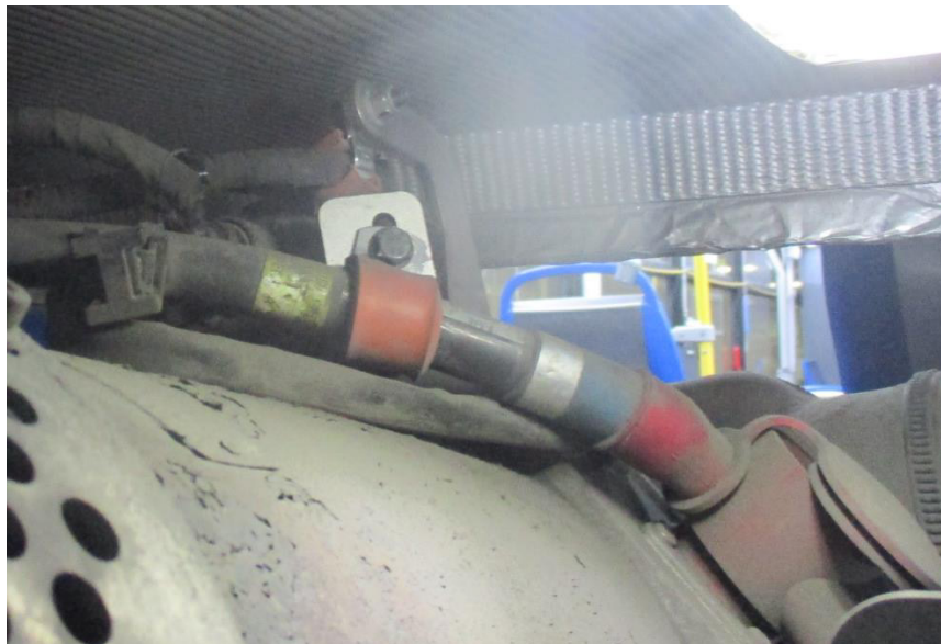
Figure 12 - Installation of P-clamp to the Alternator
