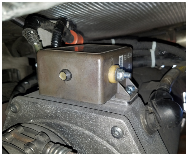
Figure 5 - Installation of P-clamp
