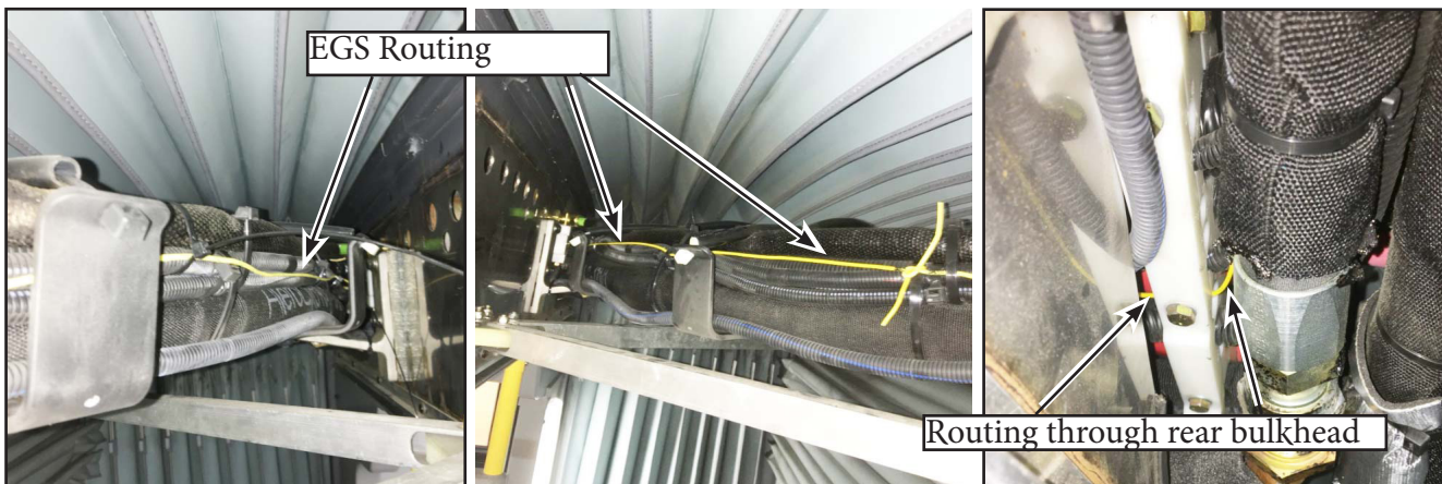
Figure 24 - Front-to-Back Cable Routing in the EGS
