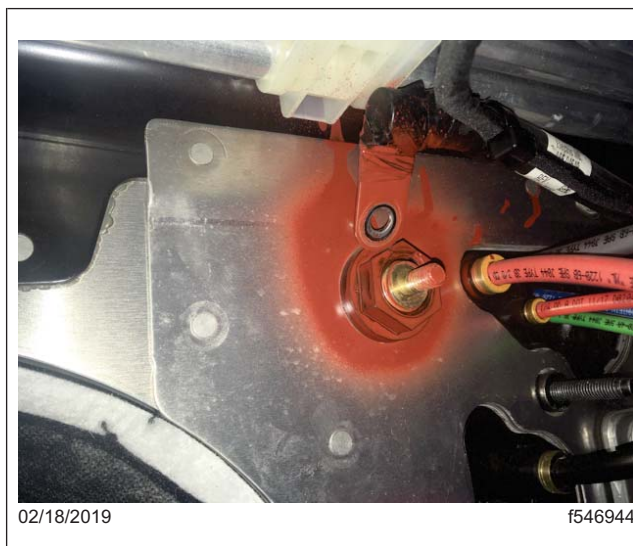
Fig. 5, GNDE Engine-Side Pass-Through Stud
