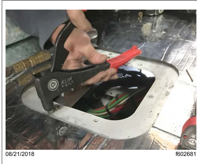
Fig. 3, Riveting the Floor Support to the Sides of the Opening
