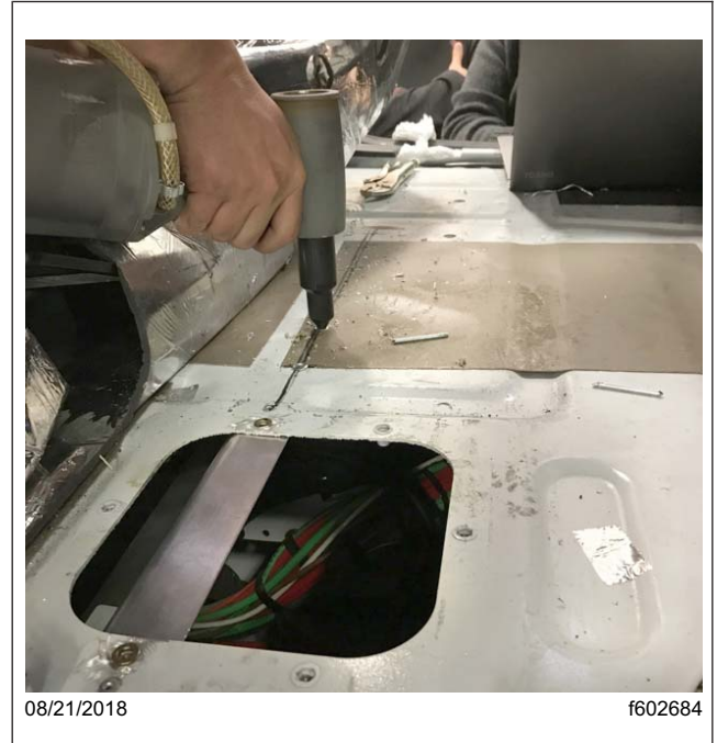
Fig. 4, Riveting the Floor Support to the Cab Floor
