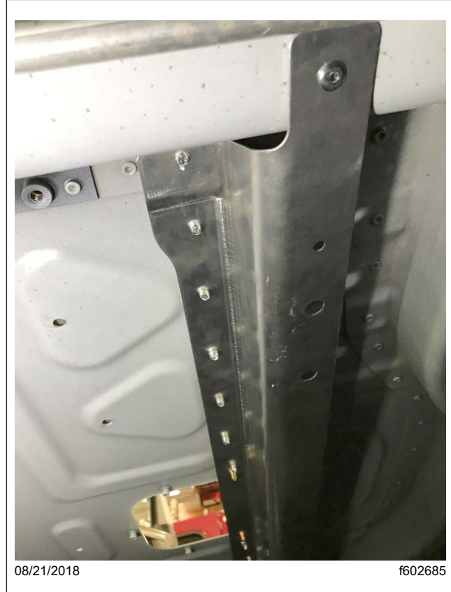
Fig. 6, Floor Support Attached to the Cab Floor and Frame
