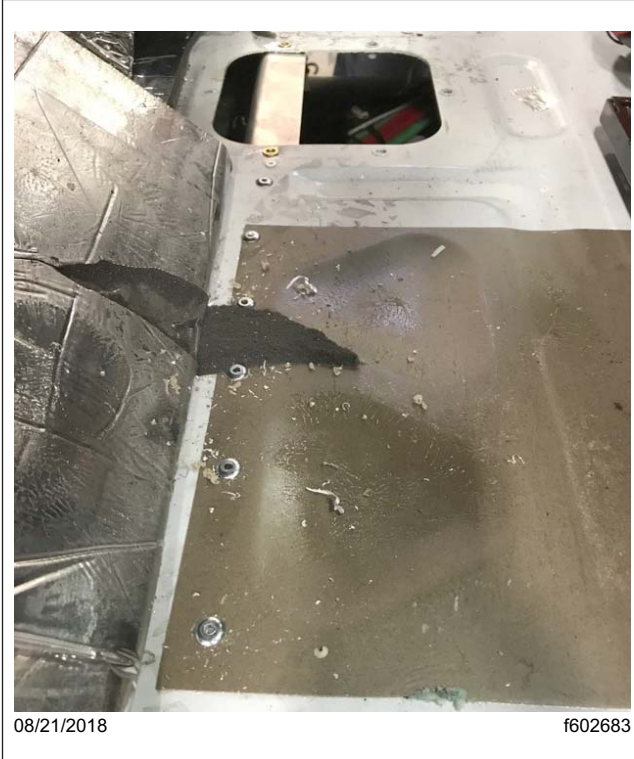
Fig. 5, Floor Support Riveted to the Cab Floor
