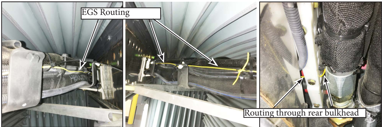
Figure 24 - Front-to-Back Cable Routing in the EGS
