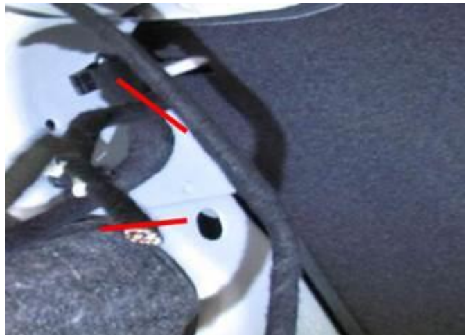
Figure 14. Open the winding of the cut-off vehicle wiring harness to the junction of the main harness on the separable area (red marks).
