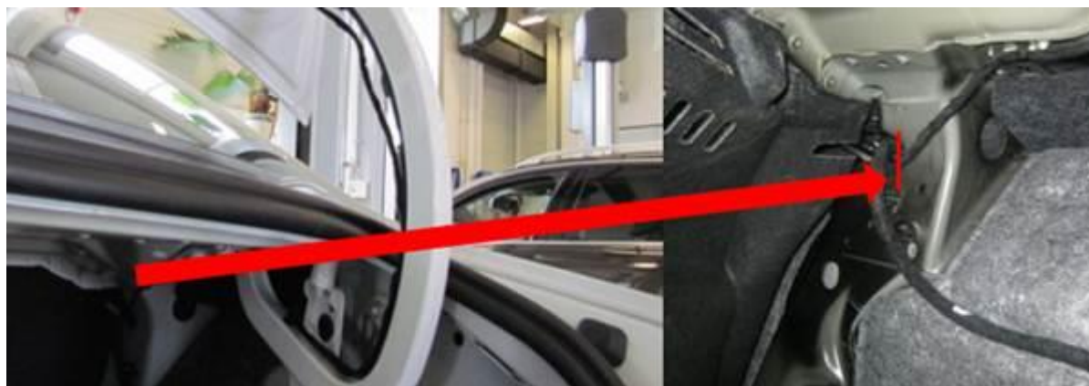
Figure 5. Cut cable off on the junction of the main wiring harness (red separation line).
