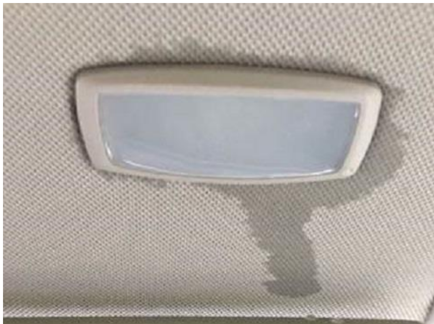
Figure 1: Example of water leak coming from the front vanity light.
