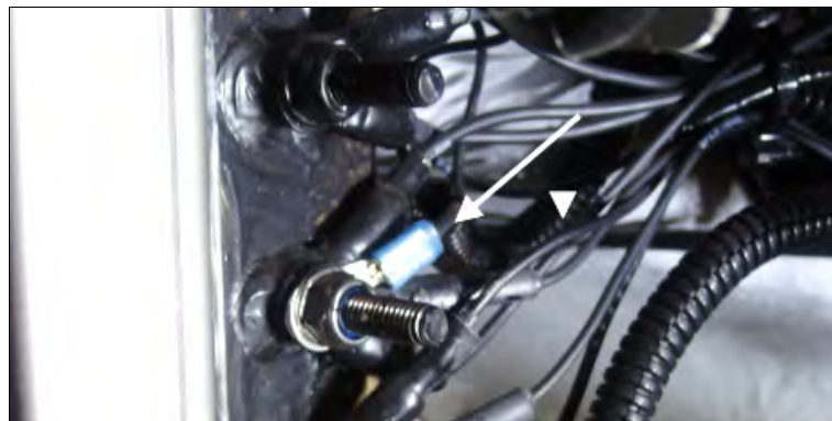
GROUND WIRE CONNECTED
