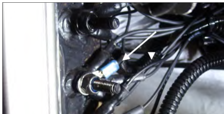
GROUND WIRE CONNECTED
