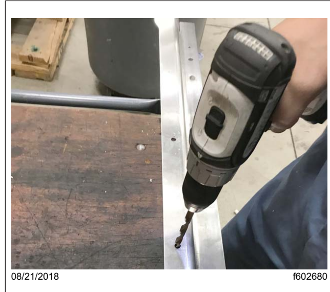
Fig. 2, Drilling Holes in the New Floor Support
