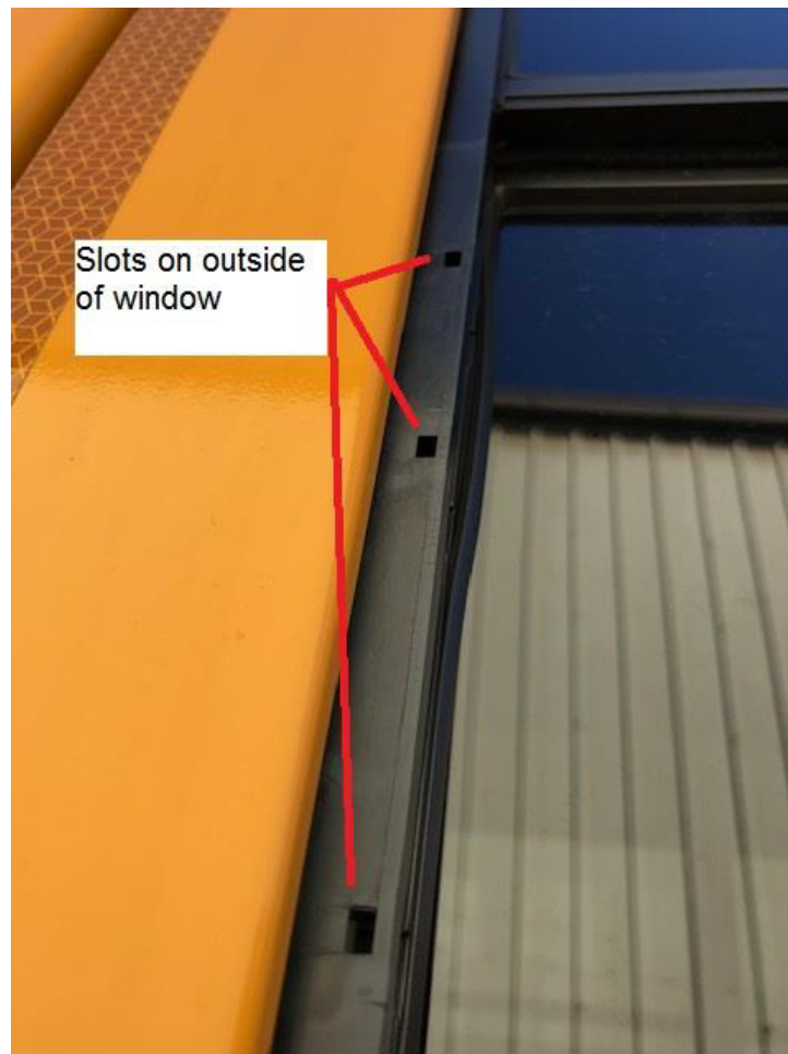
Figure 1: Locations of the slots on outside of window. (Left side shown)
