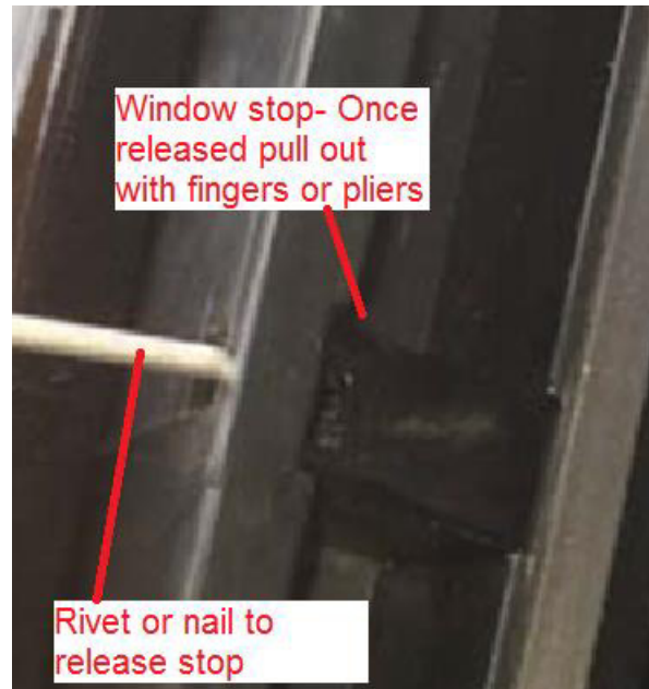
Figure 2: Location to push in with nail/rivet and how to remove stop
