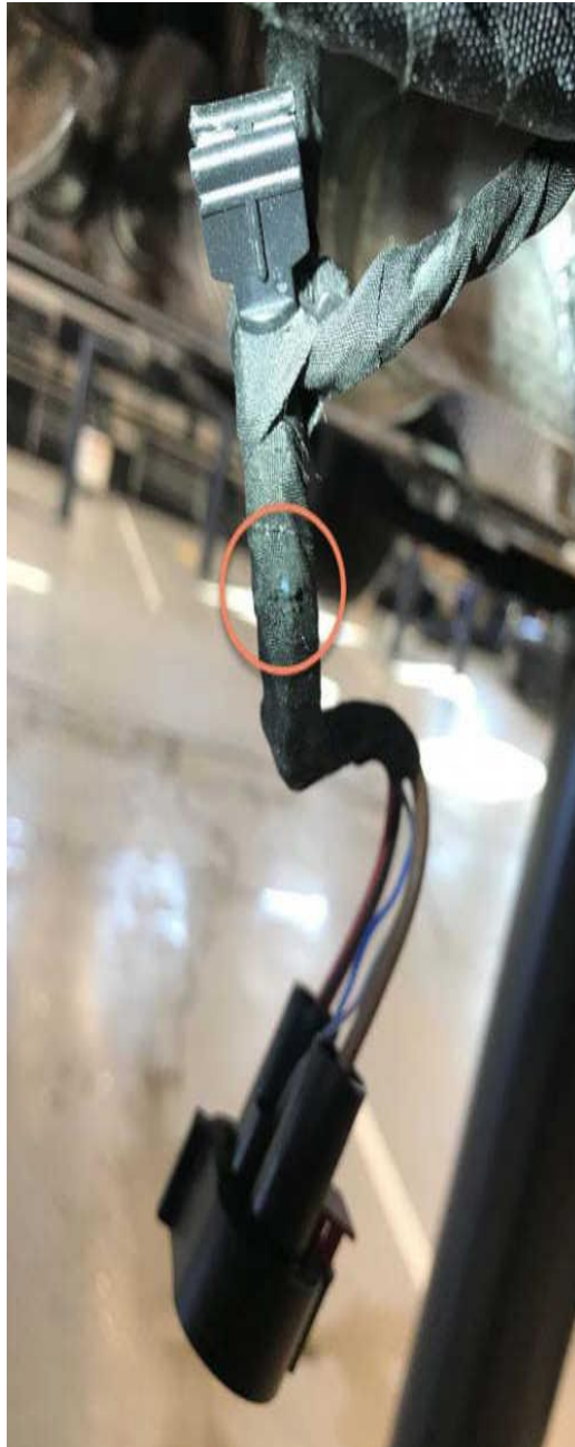
Figure 3. The damage on the harness might be difficult to spot.
