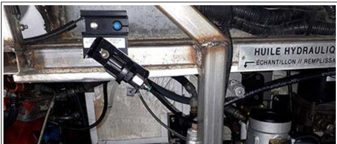
Figure 6 - Remote Breather Installed on Frame
