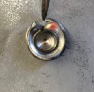
OK Rivet with 1 crack
