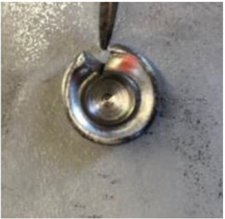
OK Rivet with 1 crack
