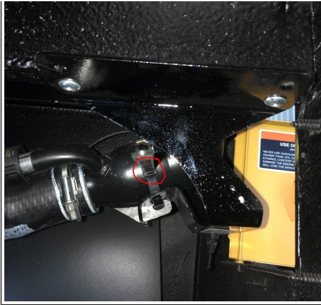
Figure 4 - Acceptable Fuel Fill Hose Droop
