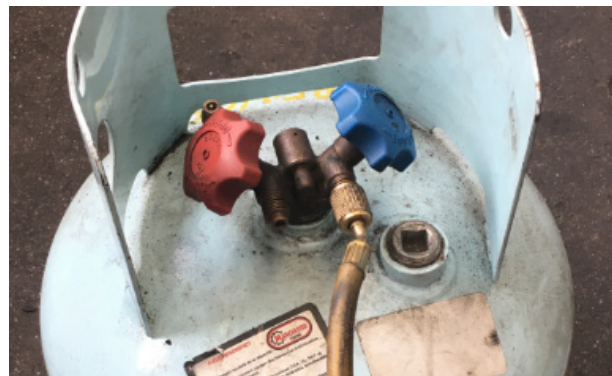
FIGURE 7: TANK CONNECTION (LIQUID)
