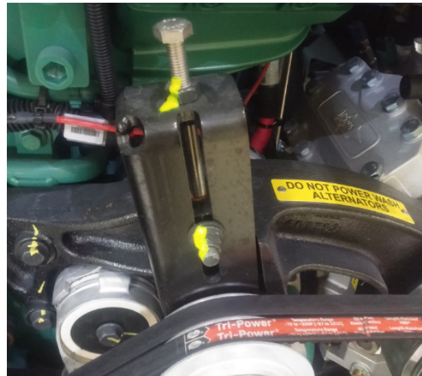
FIGURE 55: TORQUE SEAL ON INSTALLED AND ADJUSTED BELT TENSIONER
