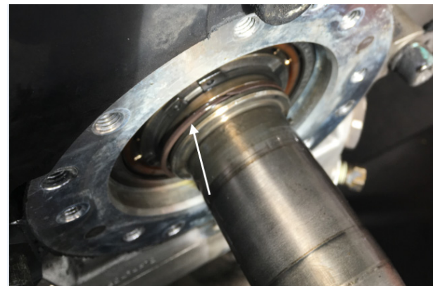
FIGURE 30: NEW RADIAL GASKET RING IN PLACE
