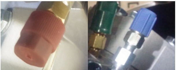
FIGURE 65: PROTECTIVE CAPS ON HIGH & LOW SERVICE PORTS
