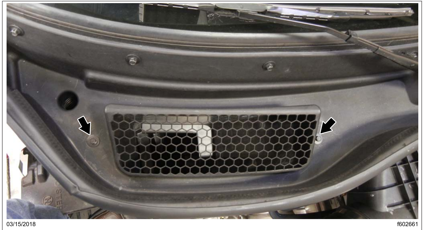
Fig. 3, HVAC Air Intake Fasteners
