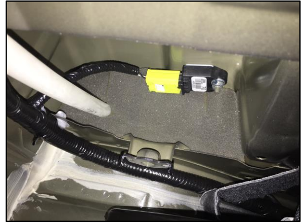
Figure 3. No. 5 Pillar Pad Installed
