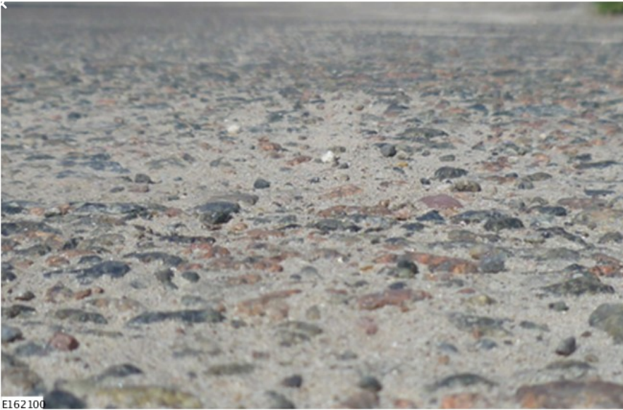
Typical road surface that can generate the rattle sound.
