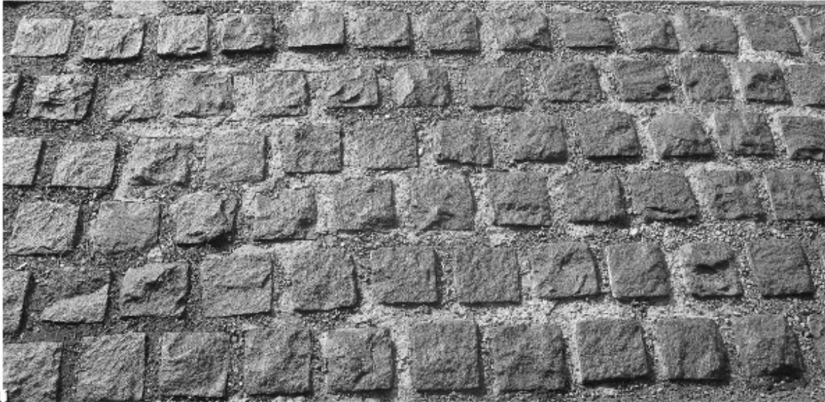
Typical road surface that can generate the rattle sound.
