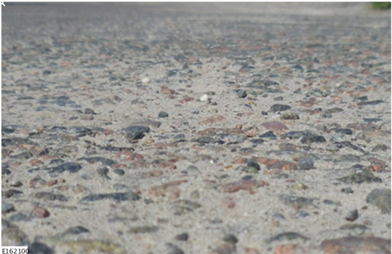
Typical road surface that can generate the rattle sound.
