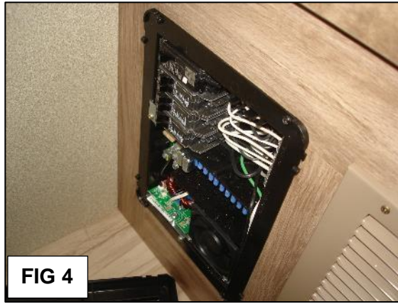
FIG 3: Remove one screw holding the cover to the breaker panel. FIG 4: Cover will pop off, revealing the breakers.
