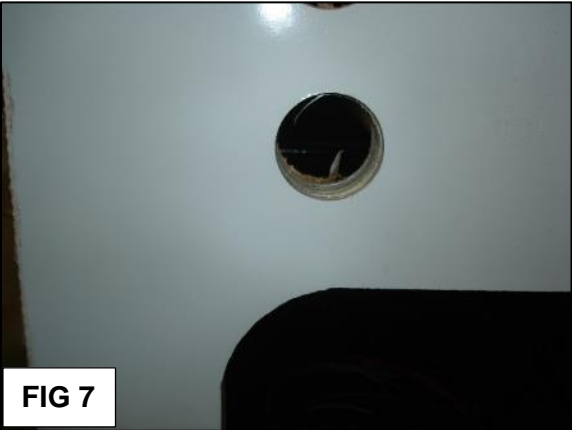
FIG 7: Drill the 2 inch diameter hole when the location has been finalized. FIG 8: While drilling, you will enter through a thick layer of wood followed by a thin layer of aluminum.
