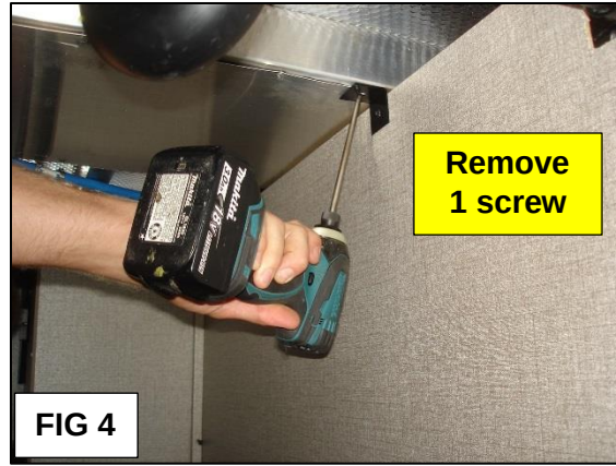
FIG 4: Remove 1 screw in the bracket at the top of the partition.
