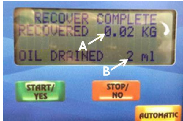
Figure 3. Amount of refrigerant recovered (A), and amount of oil drained (B).
